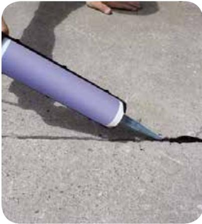
Sealing cracks and joints represents one of the most effective maintenance jobs on road and airport surfaces.
